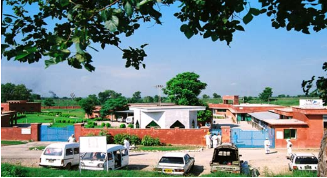
(LRBT Mandra Hospital – Front View)
