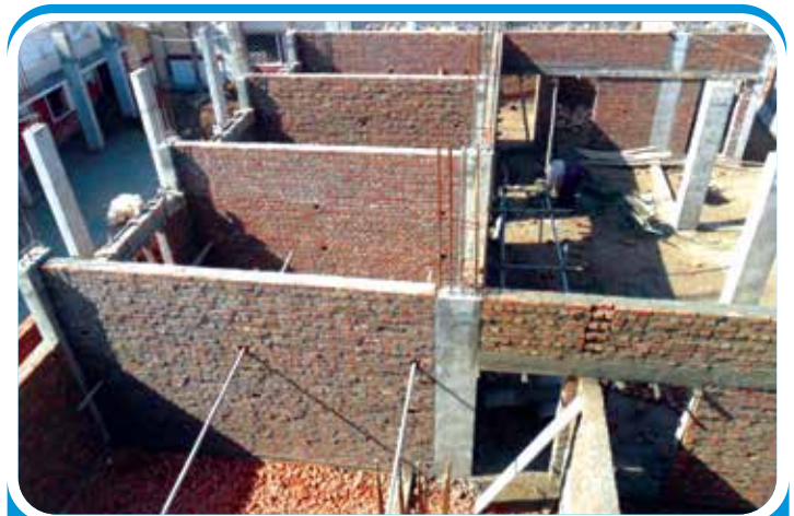
Construction of LRBT, Lar (Multan)
